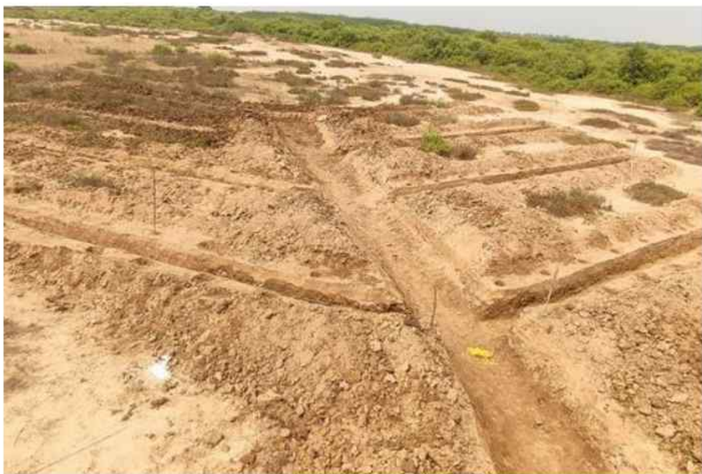
Making the path (fishbone channel) to facilitate water flow for planting saplings
