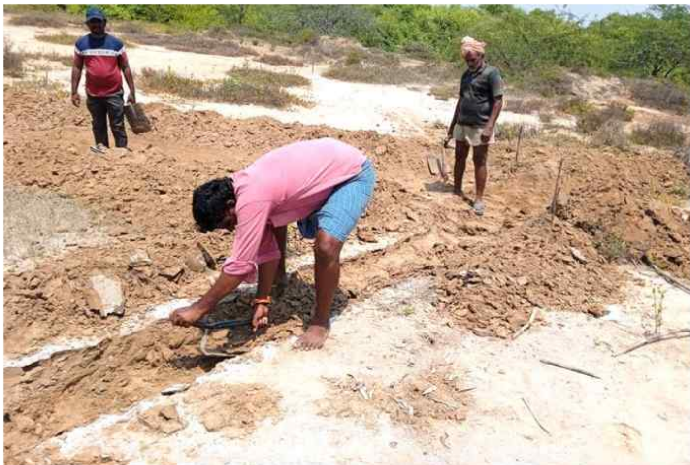
STPF members are digging the main feeder channel for water flow
