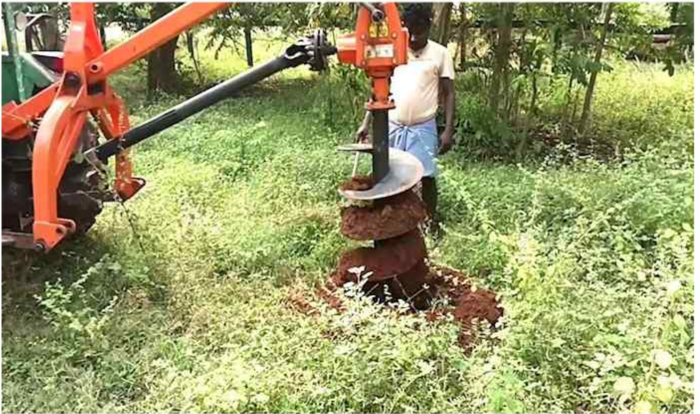
Pits (1.5 feet X 1.5 feet) being dug at the TREE Foundation, Kurumburam Biodiversity Education Center
